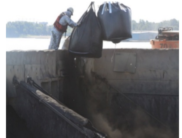
Placement of activated carbon into a barge of mechanically dredged material.
