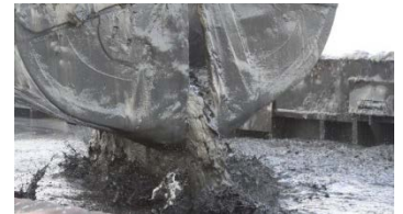
Mixing of dredged material with activated carbon in dump scow.
