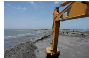
Berm construction in Louisiana
