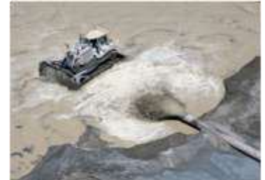
Figure 1: Placement of dredged material for beneficial use at Hamilton site
