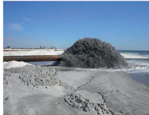
Figure 2. Beneficially using material dredged from the navigation channel for placement along shorelines to reduce erosion and enhance environmental habitat (Perdido Pass, Alabama).
