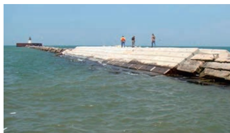
Figure 5. Habitat-enhanced toe block installation during breakwater repair operations.
