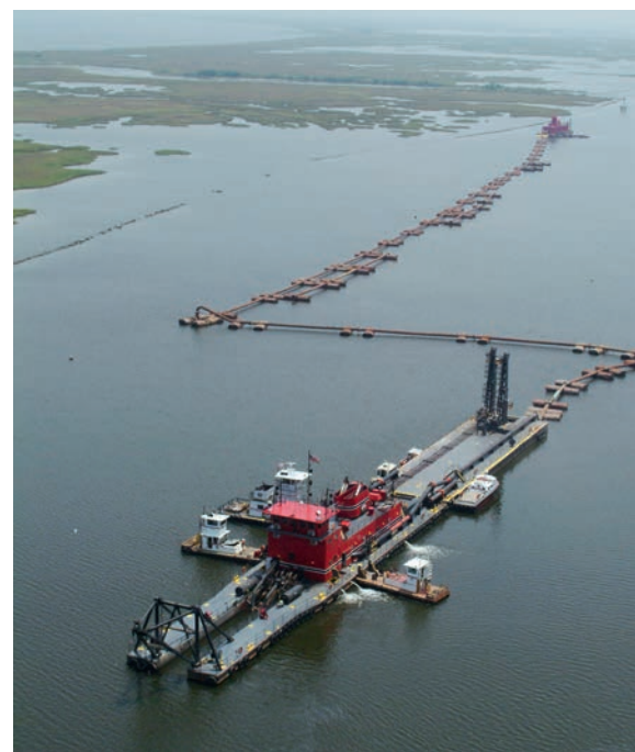
Figure 3. Long-distance pumping of dredged sediment for beneficial use and wetland restoration on the Gulf Coast.
