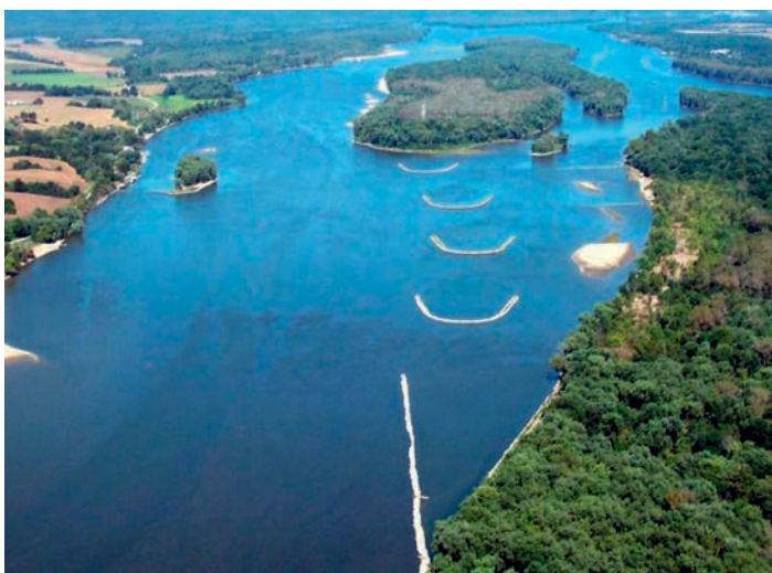
Figure 8. Chevrons at Bolter's Bar on the Mississippi River help maintain the location of the navigation channel while preserving secondary channels for habitats.
