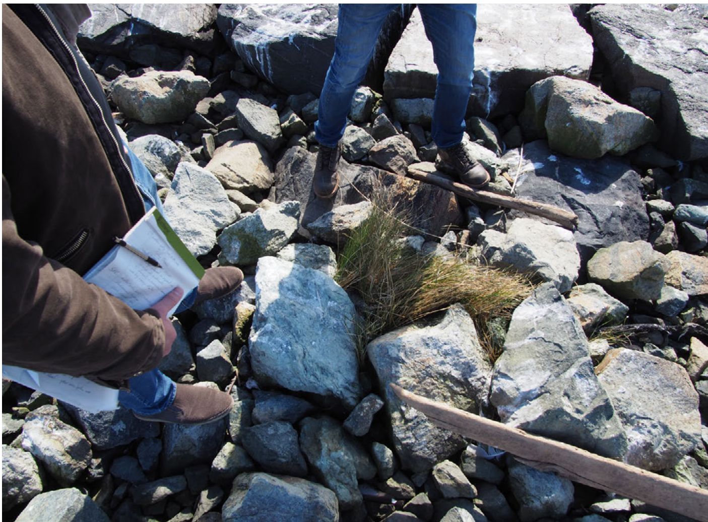
Fishing Creek North Jetty Project team members inspect existing conditions in October 2018
