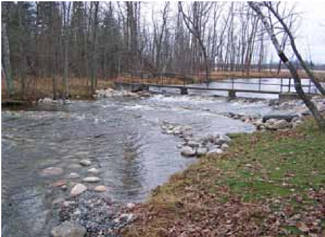
Figure 14. Rock arch rapids used to replace a low head dam (Photo courtesy of Minnesota Department of Natural Resources).
