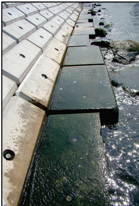
Figure 4. Cleveland Harbor breakwater constructed of concrete toe blocks (partially submerged and algae covered) and slope blocks (photo: T.J. Fredette).
