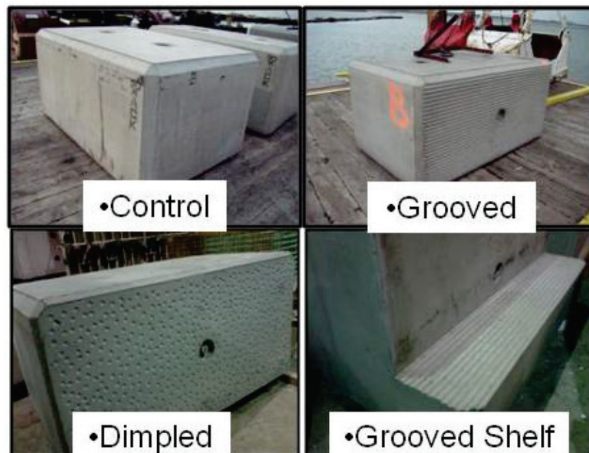
Figure 5. Control and modified toe blocks used in the Cleveland breakwater repair (photos: T.J. Fredette).
