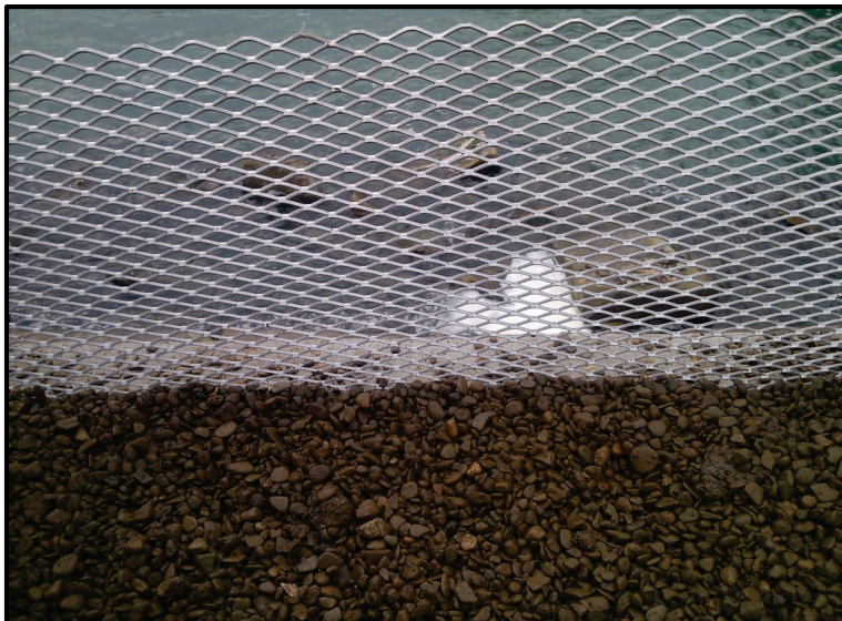
Figure 5. Pea gravel and stainless steel mesh fencing installed on the nesting habitat blocks.
