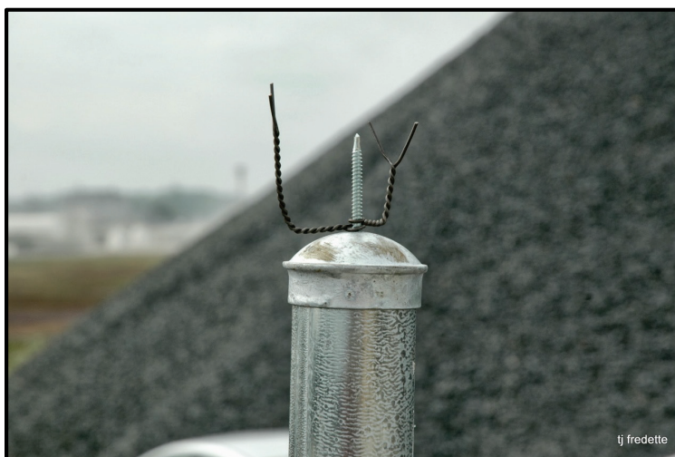
Figure 8. Gull roosting deterrent spikes on fence post caps.
