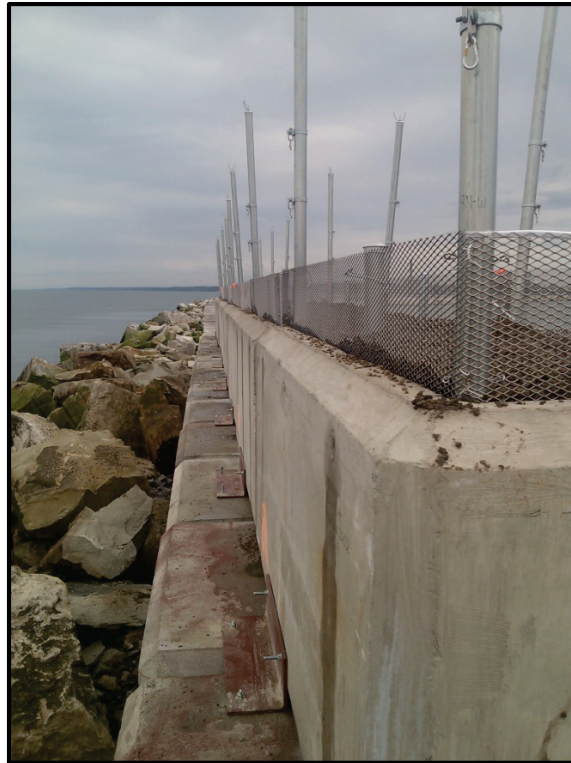
Figure 4. Angle iron cleats installed at the base of the habitat blocks to increase structural stability.
