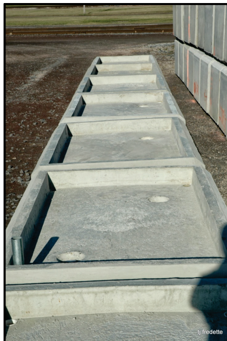
Figure 3. Modified toe blocks used for the tern habitat with top recess for nesting gravel.
