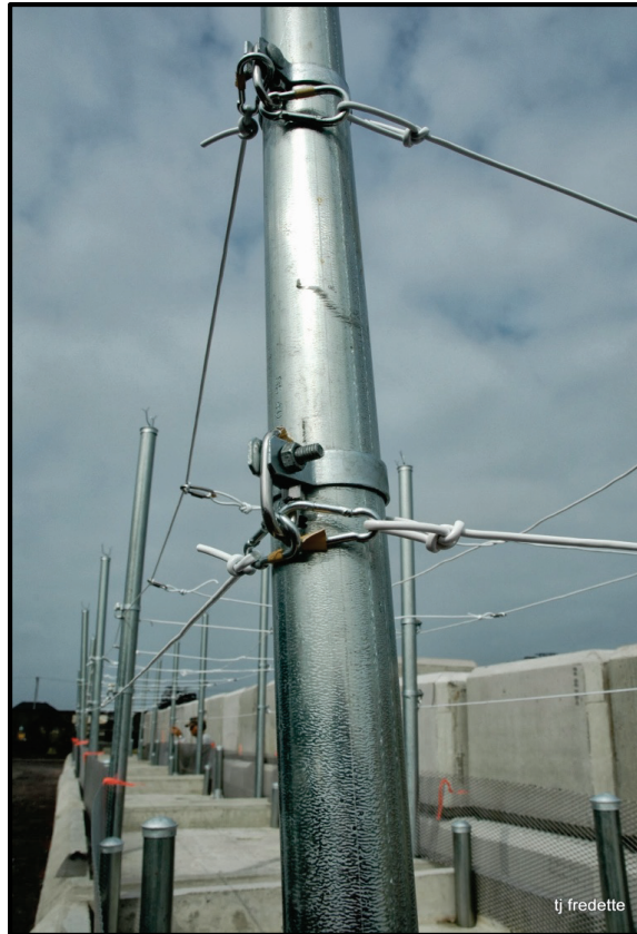
Figure 7. Carabineers and links used to attach the cabling for easy assembly and disassembly.
