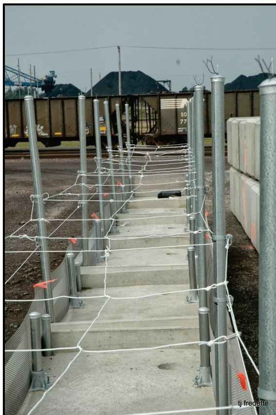
Figure 6. Predator/competitor exclusion cables. Cabling was measured, cut, and installed when the habitat blocks were still onshore. Once the installation was completed, the cable was removed for winter storage and subsequently reinstalled in spring.
