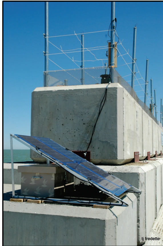
Figure 10. Solar powered tern-call system installed on the breakwater. Cables from the system power drum-shaped speakers located on each end of the habitat area.
