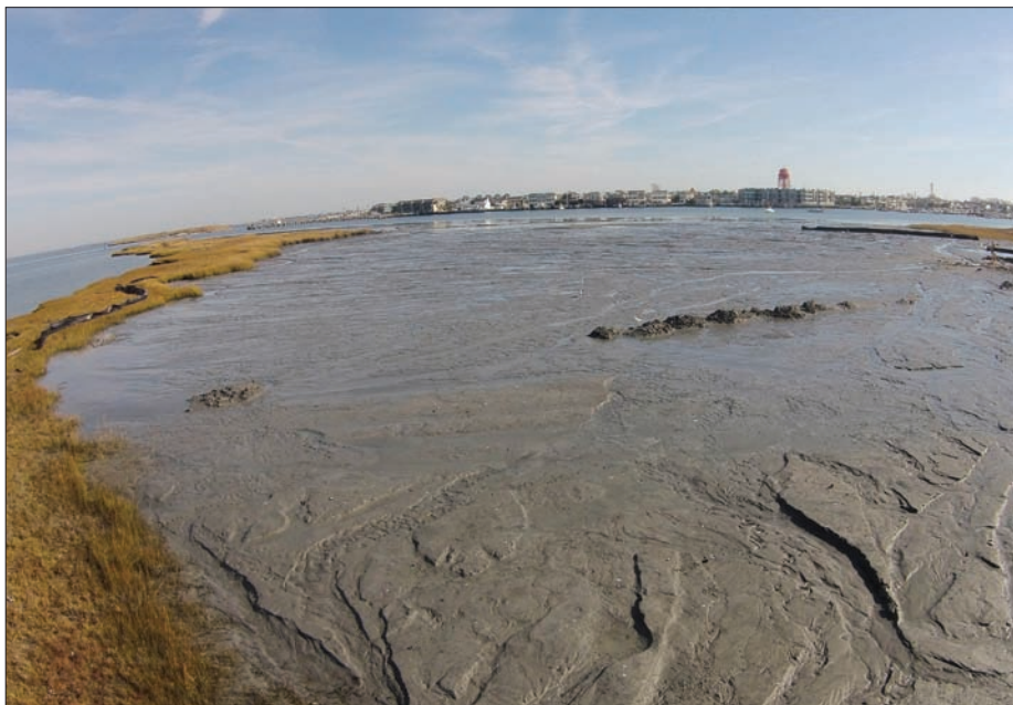
A dredging and marsh restoration demonstration project on Mordecai Island near Long Beach Island, N.J., is using dredged material from a shoal in the New Jersey Intracoastal Waterway to restore the eroded area and elevate the adjacent marsh. Planting of the restored area will be done in spring 2016. USACE PHILADELPHIA DISTRICT BY TIM BOYLE
