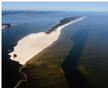
Figure 5. Left, west end breach filling, showing borrow site.
