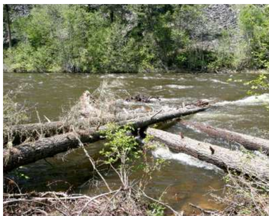
This constructed feature creates a velocity refugia and overhead cover for fish, in addition to protection of one bank, while leaving a wide path for recreational boaters. Rock Creek, Montana.
