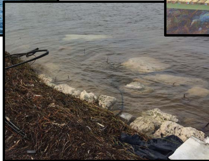
Revetment: rocks displaced
