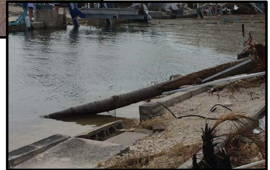
Bulkhead: cracks, undercutting, structural collapse
