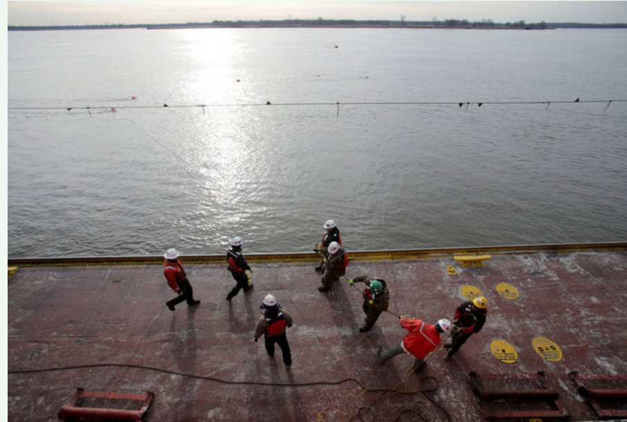
Downlines that are connected to explosives are pulled from the water by workers aboard the drillboat Apache after a morning blast off Chester, Pa., as part of the Army Corps' Delaware River deepening project, Wednesday, Jan. 20, 2016. (Tim Hawk | For NJ.com)
