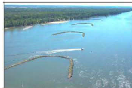
Photograph 2.13. A Series of Chevrons Aligned To Split Flow Between the Main Channel and a Side Channel, While Protecting the Existing Shoreline
