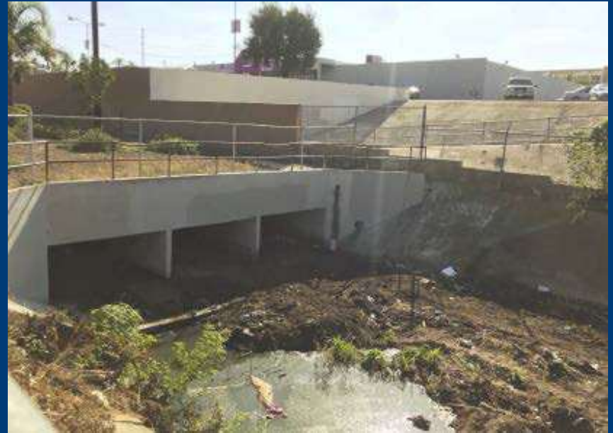
Paradise Creek after flooding receded, scouring of channel banks
