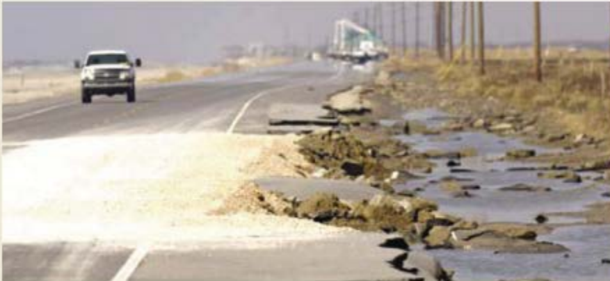
BEFORE MITIGATION: ROAD NEAR HOLLY BEACH ERODED
