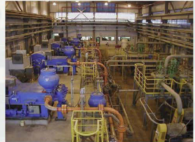
Positive Displacement Booster Pumps (source: Pipeline Systems, Inc.).
