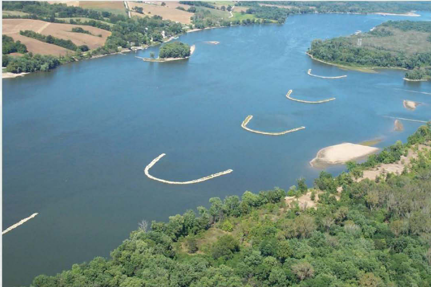
Upper Mississippi River Training Structures: Chevrons
