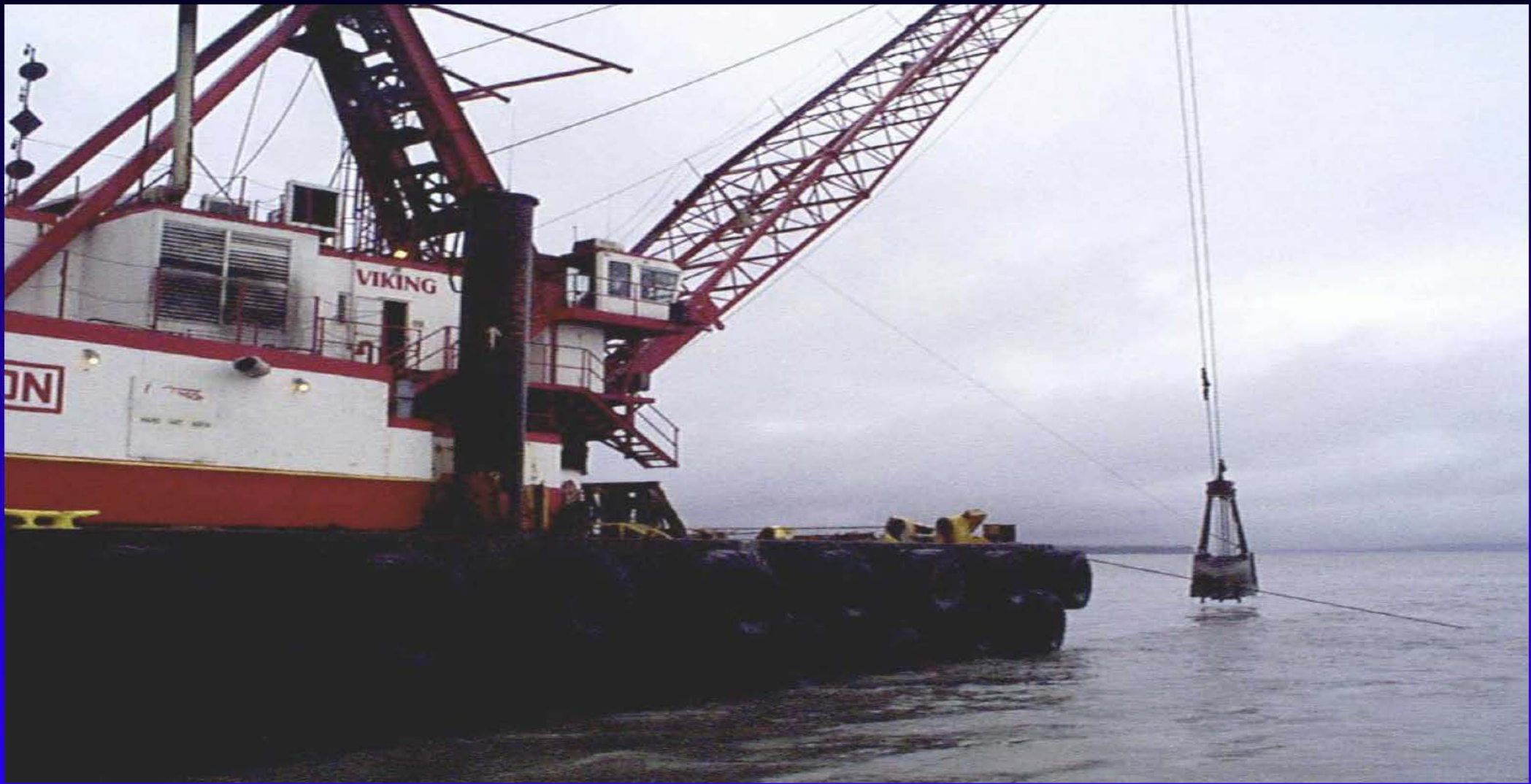
Manson Bucket Dredge Viking (1,500hp, 10cyd) Operating in Cook Inlet, Alaska
