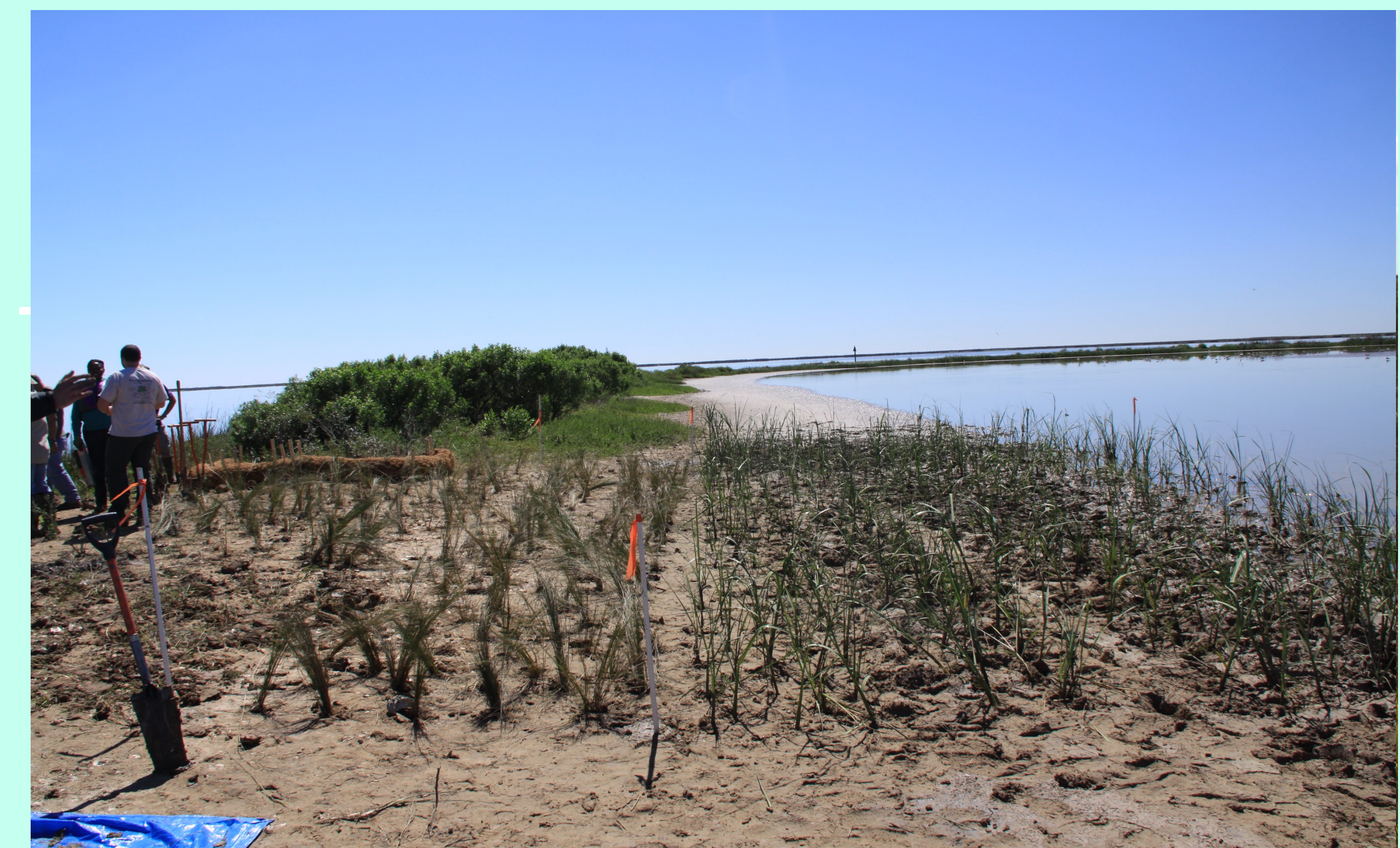
Figure 5. Completed planting of dike section.
