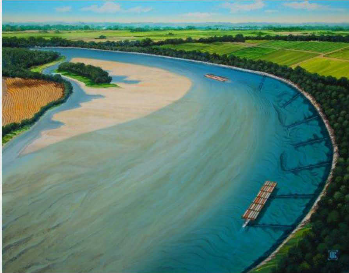
River Bendway Weirs
