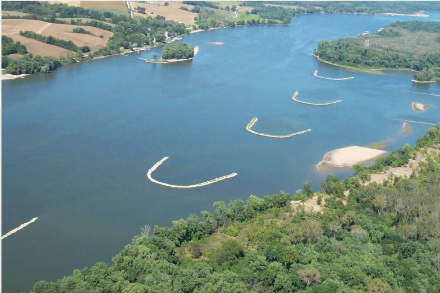
Upper Mississippi River Training Structures: Chevrons
