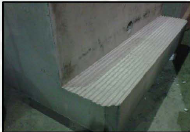
Environmentally Enhanced Breakwater Toe Blocks
