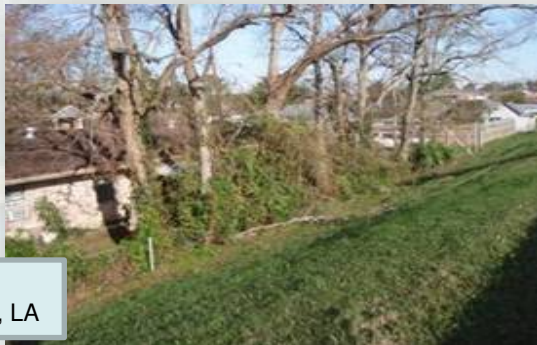
Woody Vegetation on Levees
