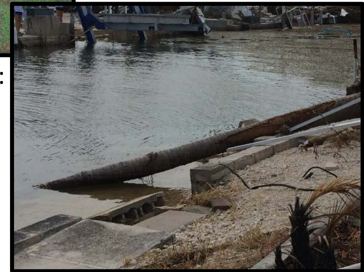
Bulkhead: cracks, undercutting, structural collapse
