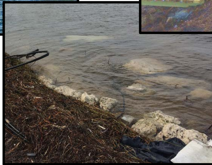
Revetment: rocks displaced
