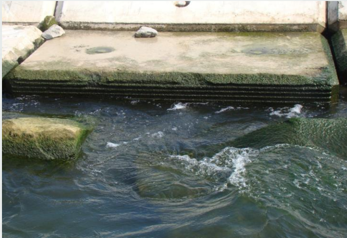
Toe block with horizontal groove (August 2012)
