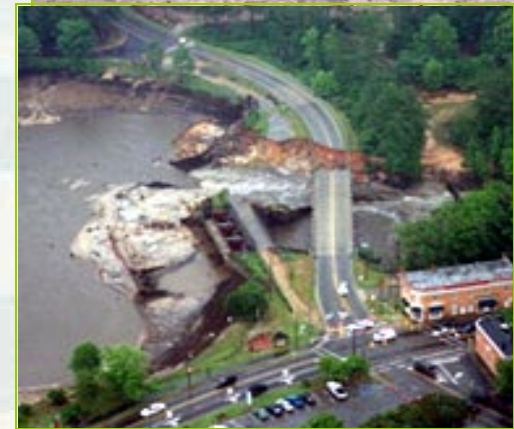
Rockfish Creek Dam failure, NC, 2003
