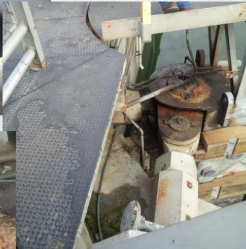
Upper pintle bearing showing grease lines
