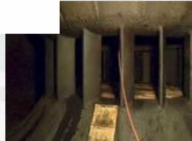
Picture of open wicket gates at Parker Dam (CA)
