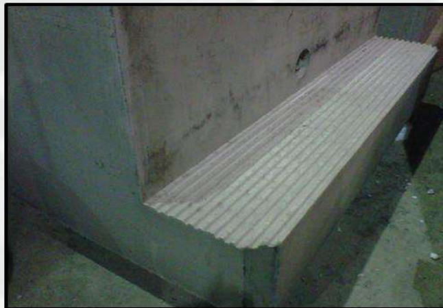
Environmentally Enhanced Breakwater Toe Blocks
