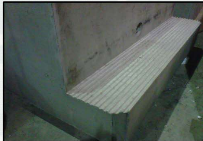
Environmentally Enhanced Breakwater Toe Blocks
