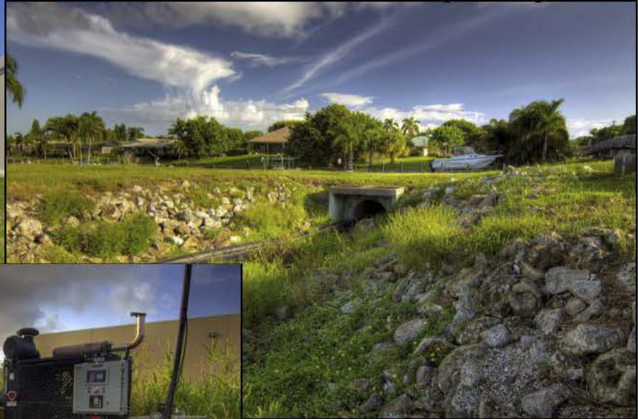
Existing Drainage Swale
