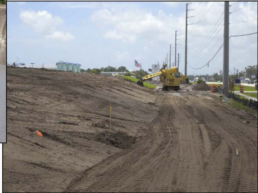
Temporary Seepage Swale
