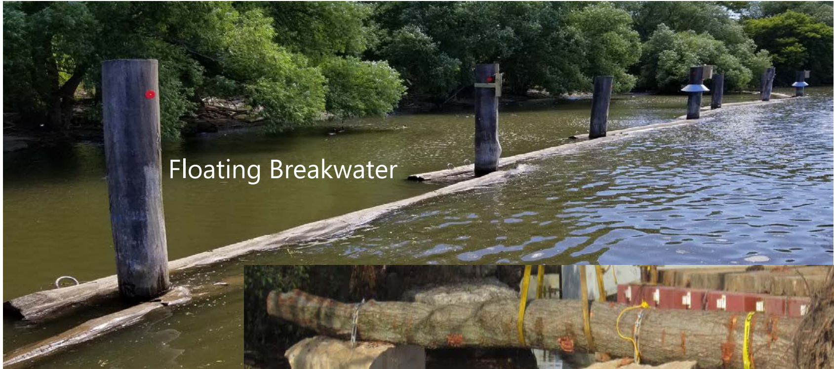
Anchored Rootwad Logs
