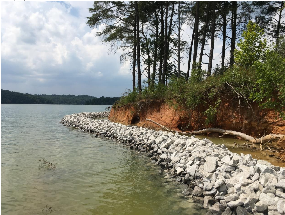
Post-project site conditions with bank erosion protection
