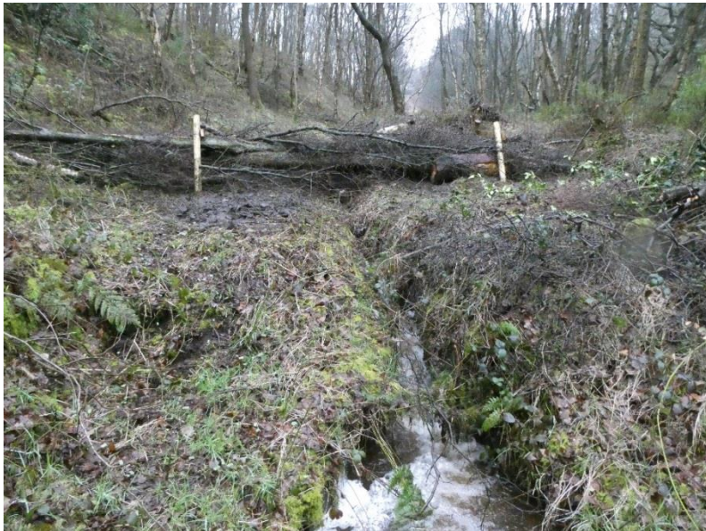
Figure 3 Leaky Barrier Built in Bradford
