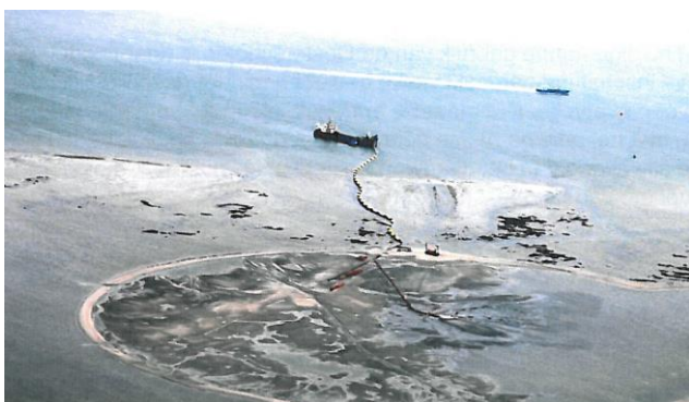
Sand nourishment under construction
