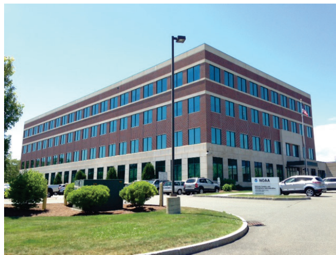
Figure 1. NOAA's GARFO Building in Gloucester, Massachusetts.
