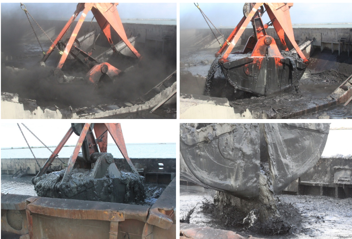
Figure 3. Mixing the activated carbon into the dredged material.
