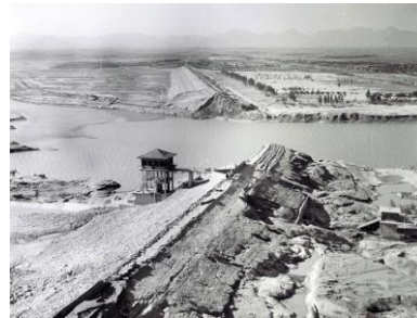
Banqiao dam failure; China, 1975
