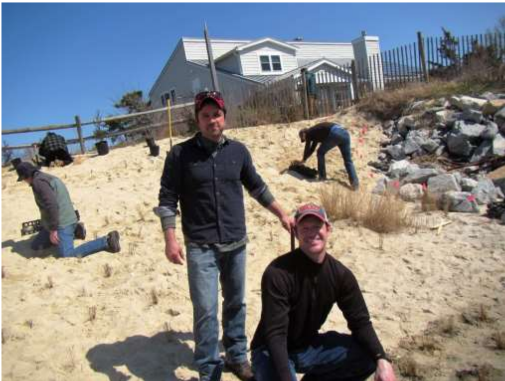
Philadelphia District engineers planting Spartina alterniflora to stabilize dunes as part of EWN demo workshop in Rehoboth Beach, DE.
