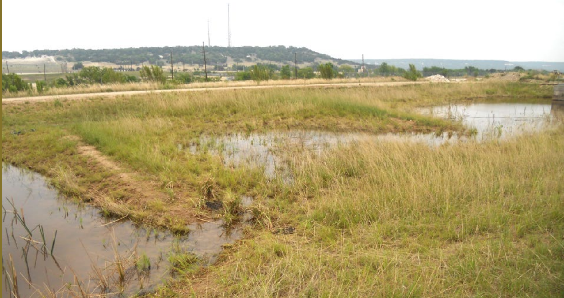
Bottom: A series of retention cells in the constructed wetland. (Photo by ERDC)
