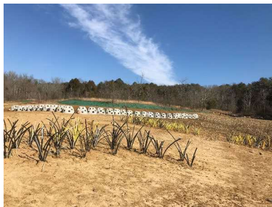
Figure 1. Nolin River Reservoir shoreline stabilization and restoration project with toe protection, reef balls, vegetative bank protection and plug plantings.
