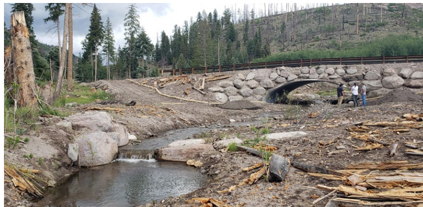
Figure 1. Santa Clara Creek stabilization and restoration project with grade control structures, vegetative bank protection and replantings, bottomless culvert design and floodplain management practices.
