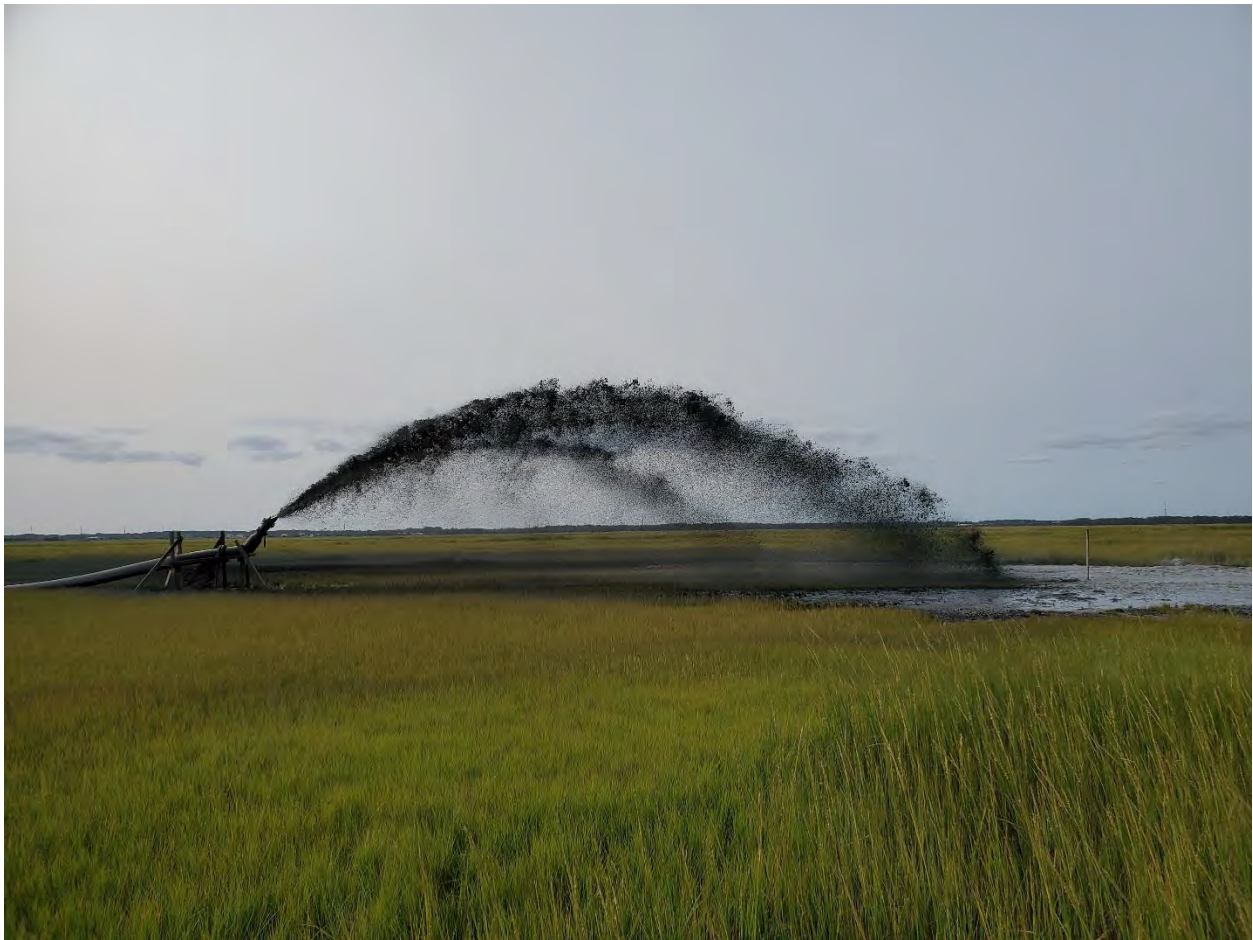
Thin-layer placement for habitat enhancement on Gull Island, NJ during navigation dredging.
