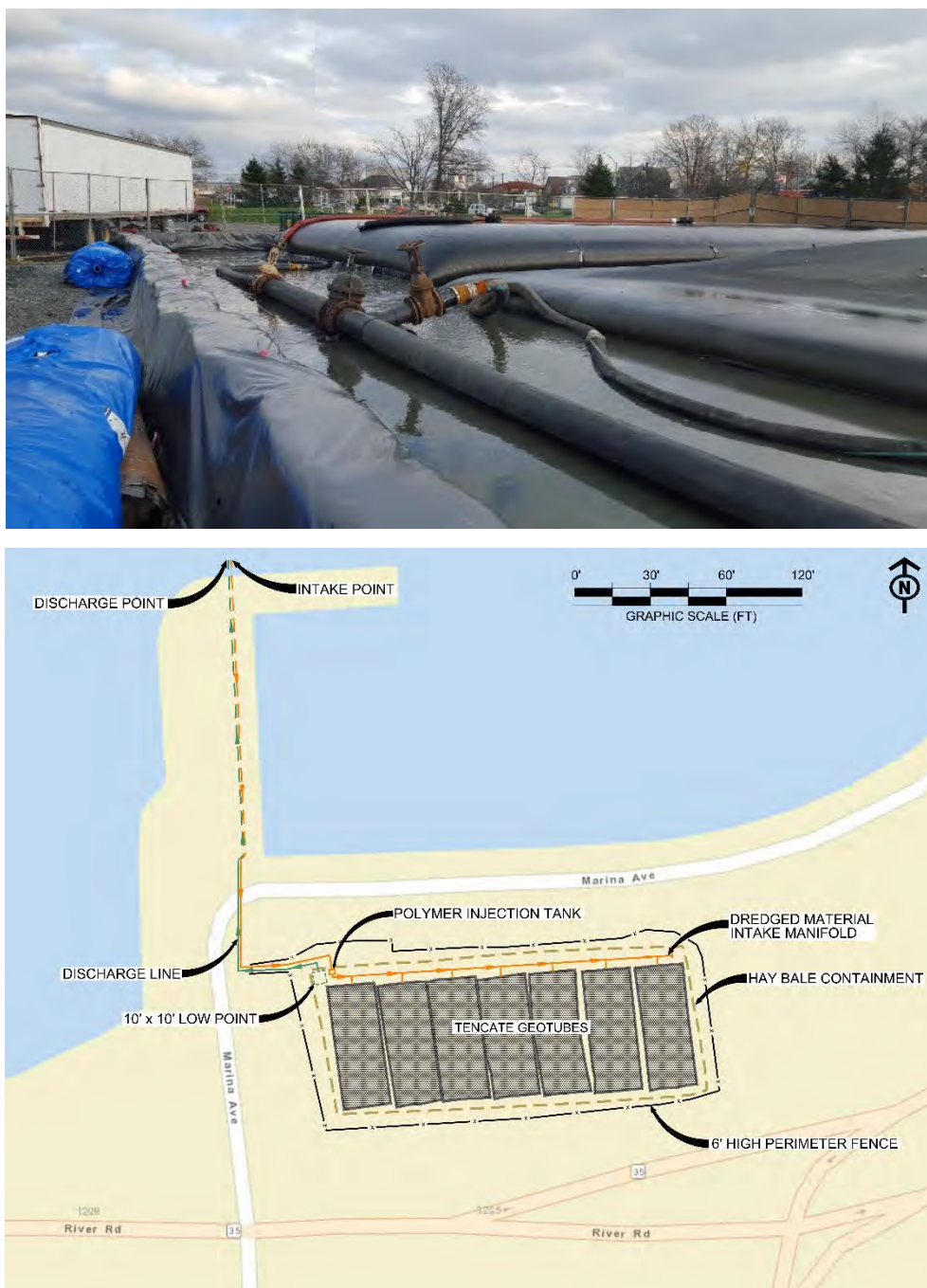
Figure 3. Site layout and photograph of Phase I passive dewatering system
