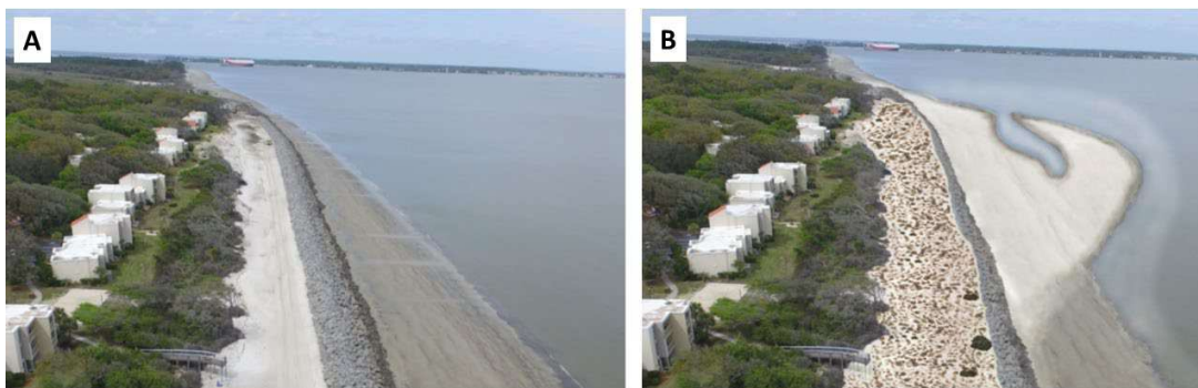
A) Northern Terminus of Jekyll Island Revetment. B) Conceptual visualization of added “sand motor” to strengthen the transition to the natural shoreline and beneficially use sandy material. In this conceptualization, vegetation has also moved into the sandy area landward of the revetment. Graphic from Hansell and Carswell (2019).
