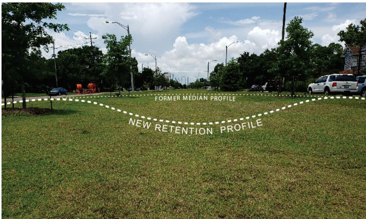
Figure 4. Ground-level view of the bioretention component of the neutral ground. Bermuda grass was planted, consistent with New Orleans Department of Parks and Parkways maintenance standards, to foster biofiltration.
