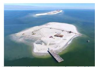
Evaluated bathymetric data, held industry days, conducted cultural surveys and allowed flexibility for start up pumping and direction of work in contract. Construct East to West or West to East or both East to West. Fill the whole template or partial template? What are the potential sediment losses?
