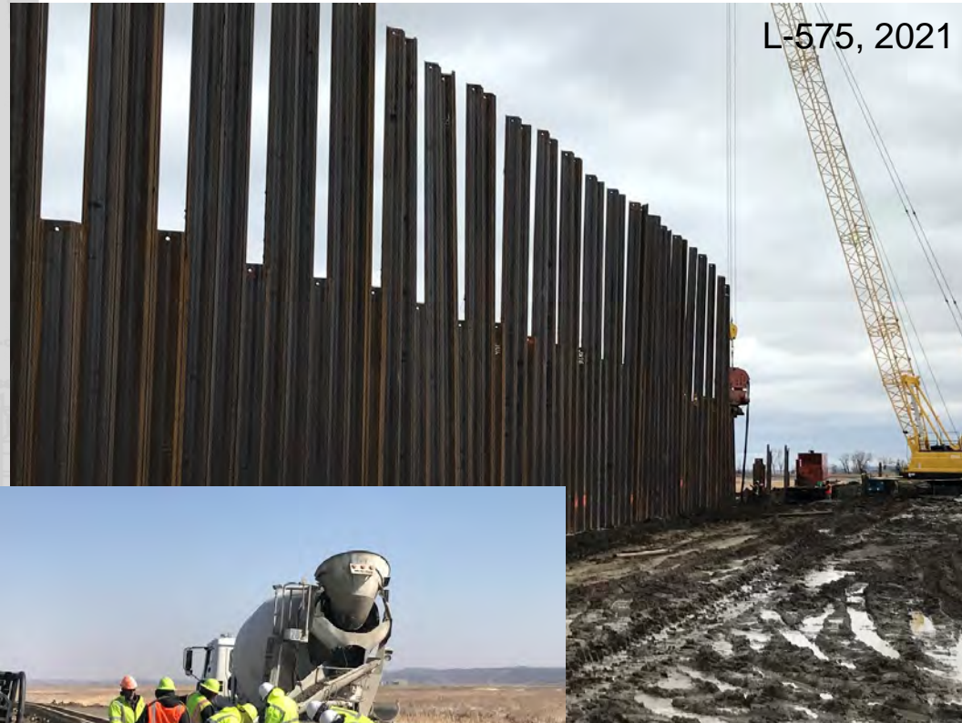
Drive miles of concrete capped sheet pile in-line
