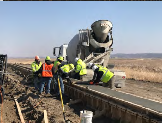
Drive miles of concrete capped sheet pile in-line
