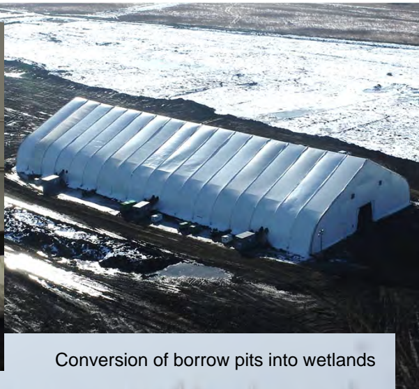
Heated tents for winter construction and material processing
