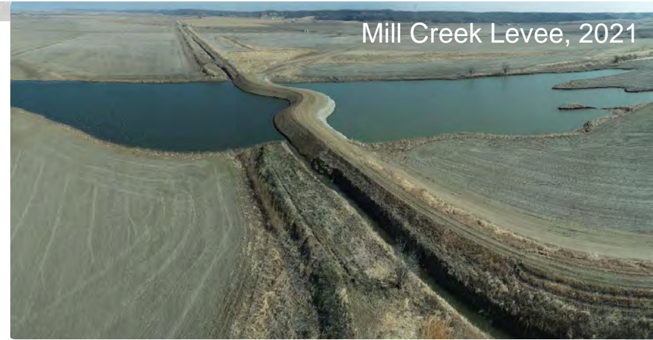
Rebuild levee through breach scour holes
