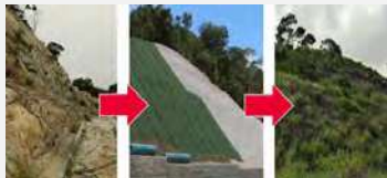
Slope Stability Aratu, Brazil
