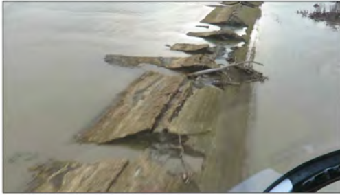
Damage on the L-536 showing breaches and water flowing through them
