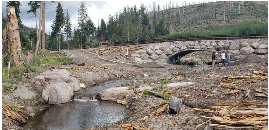
Figure 1. Santa Clara Creek stabilization and restoration project with grade control structures, vegetative bank protection and replantings, bottomless culvert design and floodplain management practices.
