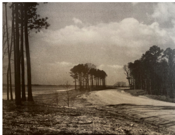
Figure 11. Parkway grading before concrete was poured, near College Creek. (1940s)
