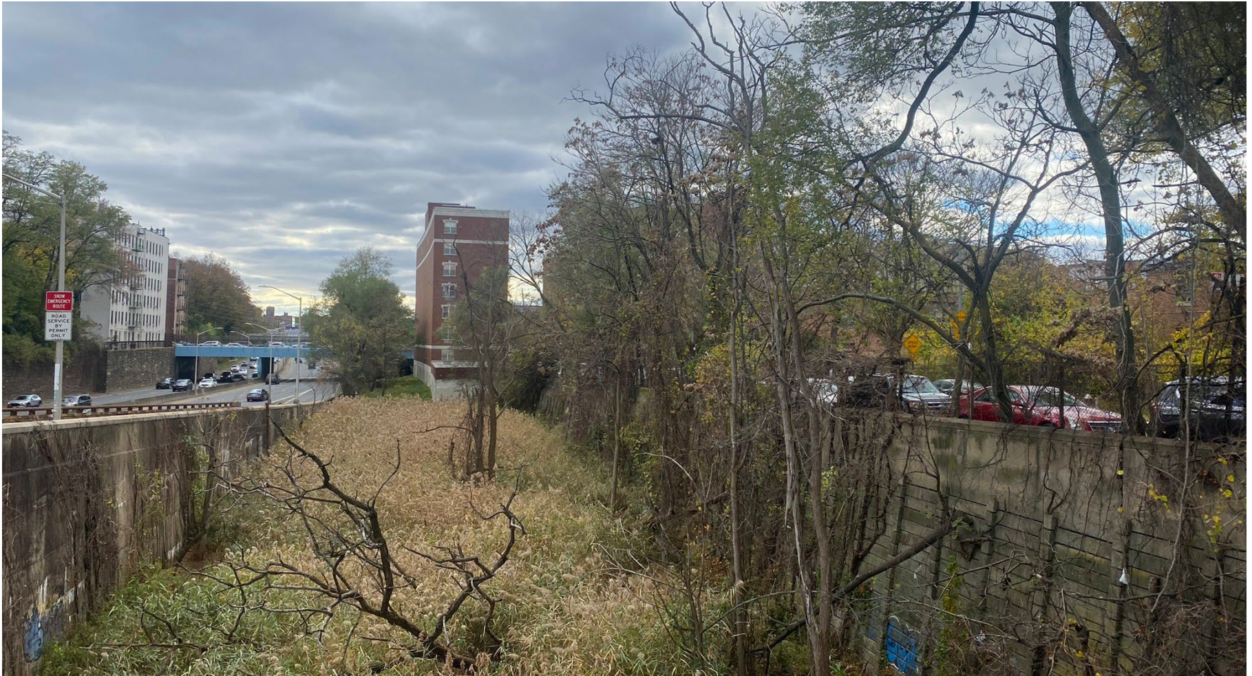
View of CSX Corridor looking South from Van Cortlandt Park South bridge
