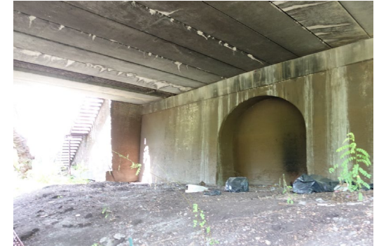
BRIDGE UNDERPASS (W. 233RD ST)
