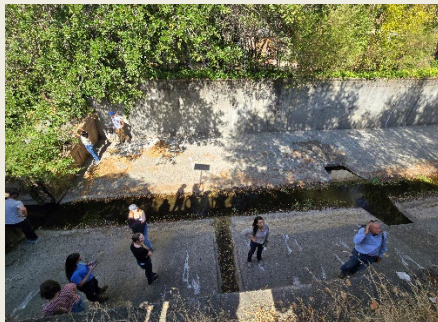
Corte Madera Creek Concrete Channel
